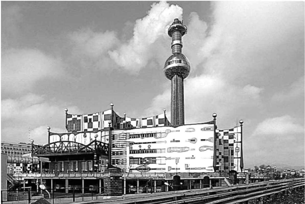
Figure 8 WTE plant Spittelau Vienna
