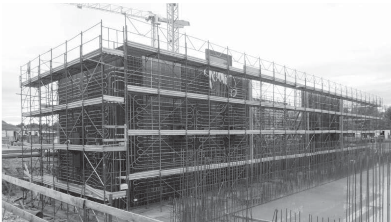
Figure 5 STRABAG LARAN ® plug-flow digester under construction (September 2014)
