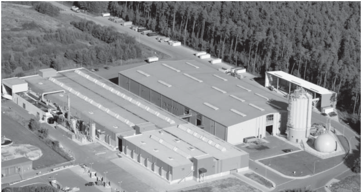
Figure 4 DRANCO installation in Hille ,Germany with partial stream digestion
