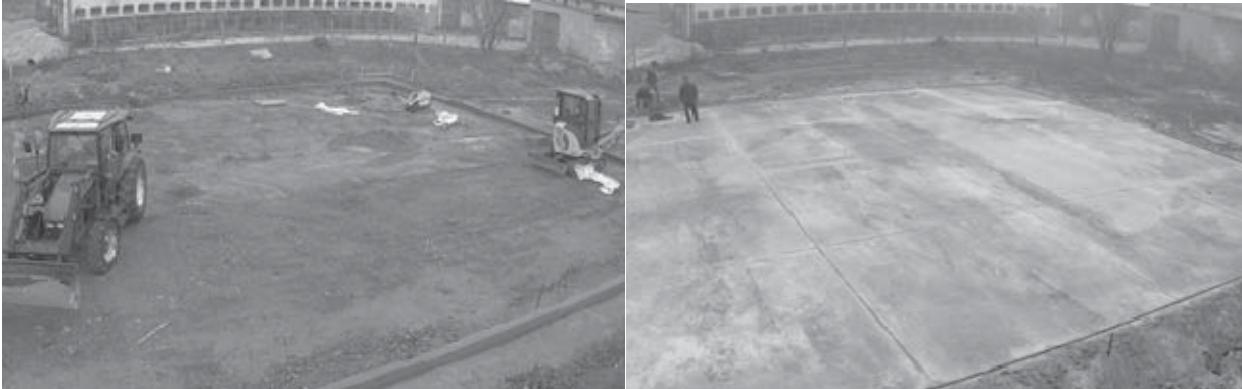
Figure 2 Construction of infrastructure; container & manipulation surface
