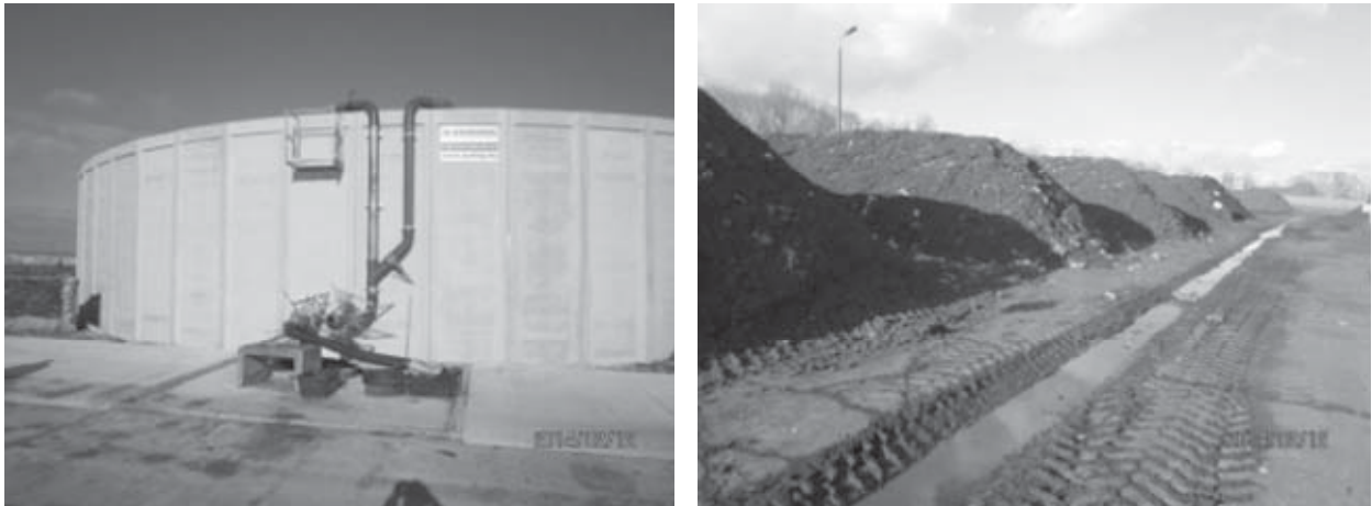
Figure 13 liquid digestate store (left, here: Milower Land, Brandenburg) and open windrow composting of solid digestate (right, here: Trappenfelde, Brandenburg)
