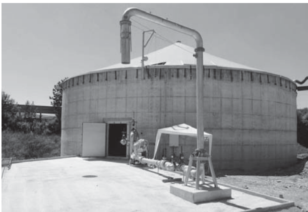
Picture 1: Liquid digestate storage tank
