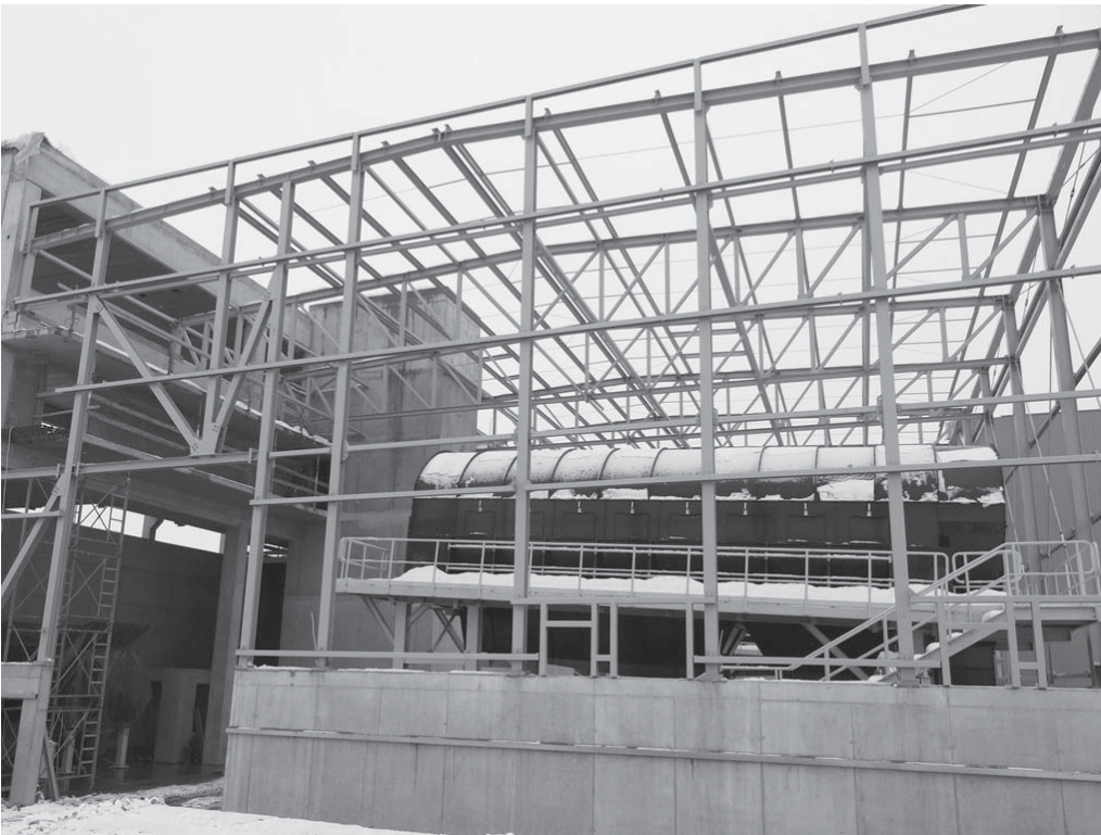
Figure 7 Drum screen for mechanical pre-treatment (January 2015)
