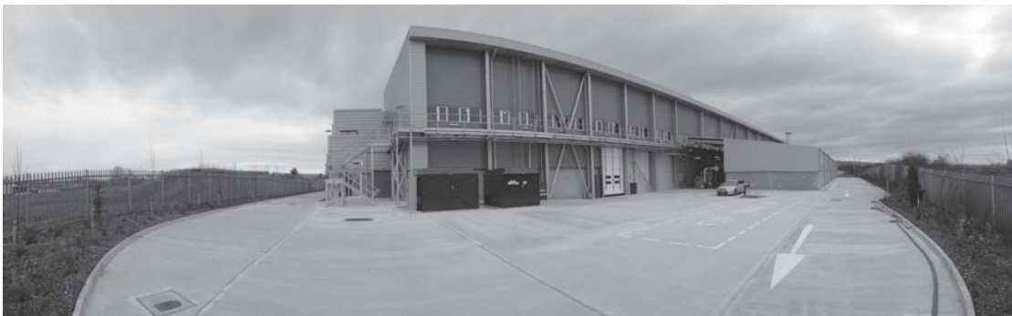
Figure 3 The Northacre RRC - Wiltshire MBT plant
