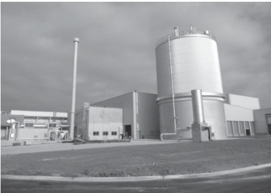
Figure 6 SORDISEP installation in Bourg en Bresse, France
