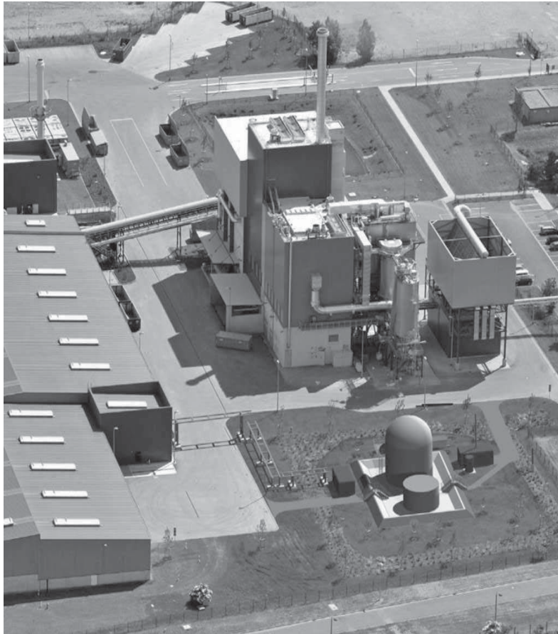
Figure 2 View of the RABA Erfurt Ost plant from the initial situation in 2008 (a photo montage of the percolate fermentation plant, then in the design stage, is included in the lower right portion of the photo).
