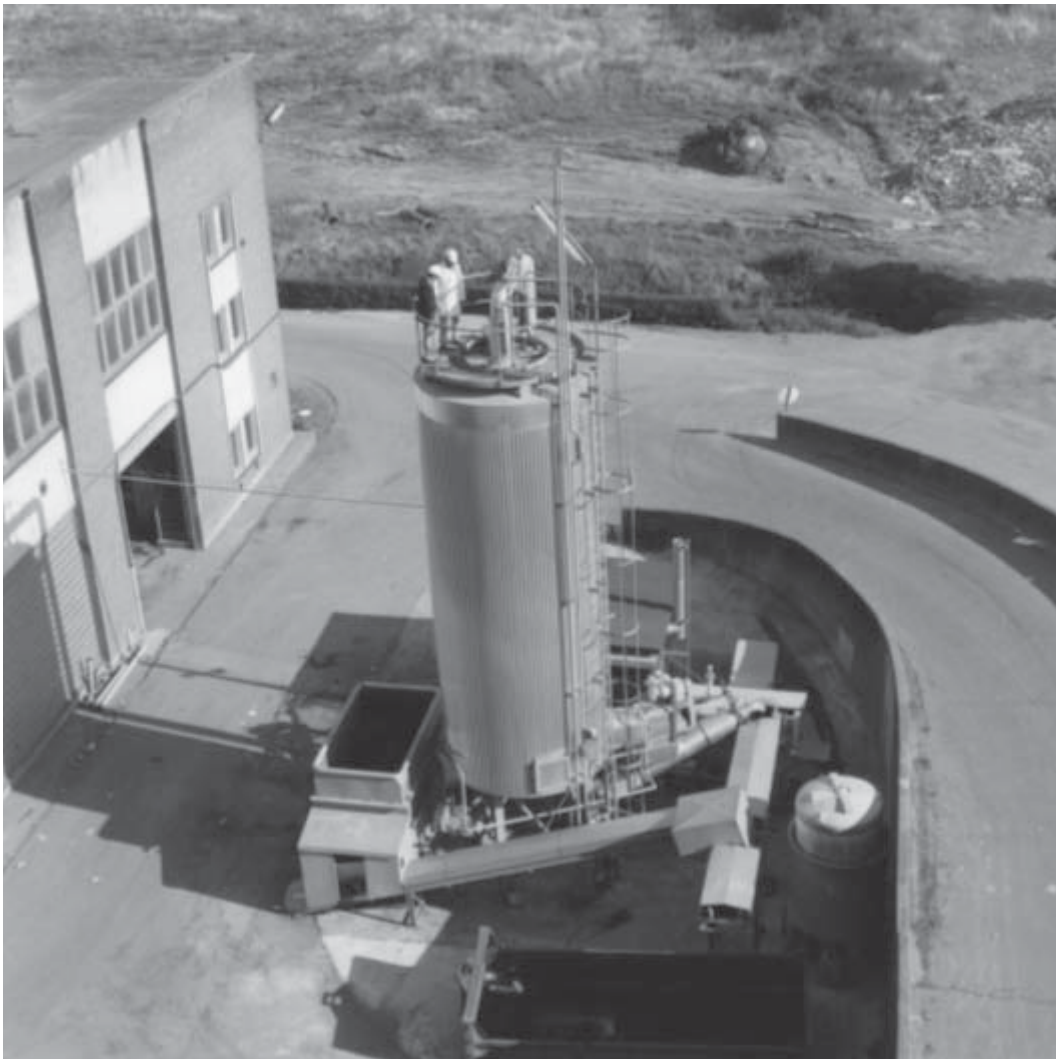
Figure 1 DRANCO pilot plant for the digestion of MSW, constructed in 1984
