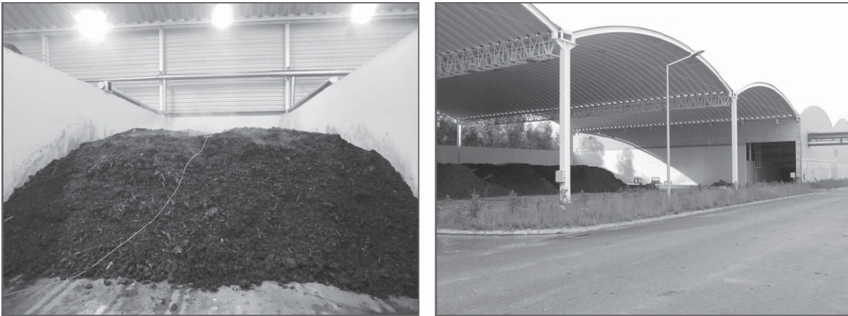
Figure 6 Composting boxes for the pre-composting phase and post-composting hall
