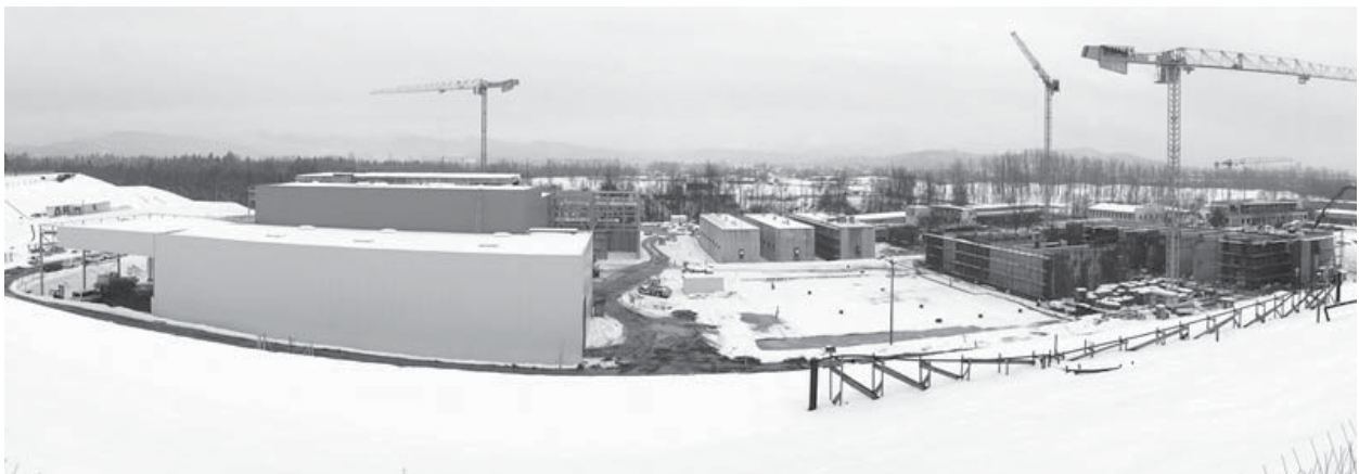
Figure 9 Scenic view on the hibernal construction site (February 2015)
