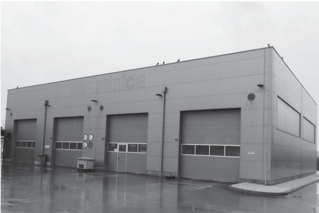
Figure 4 New car wash of RCERO Ljubljana (start-up 2013)
