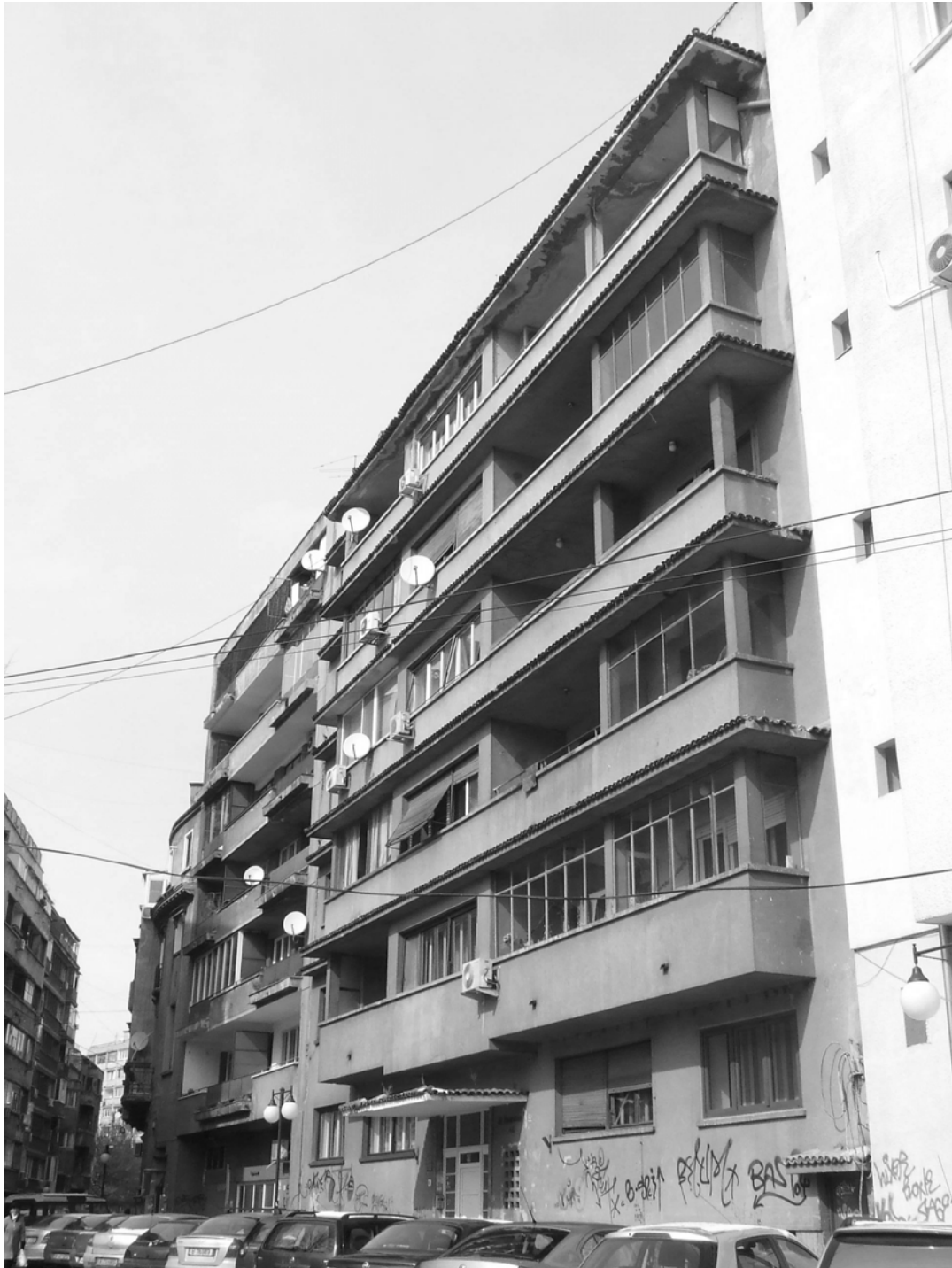
Figure 1-1: Block of flats on Brezoianu street (1946-48), architect Henrietta Delavrancea-Gibory, combining traditional and modern elements. Photo by Maria Bostenaru, 2010.
