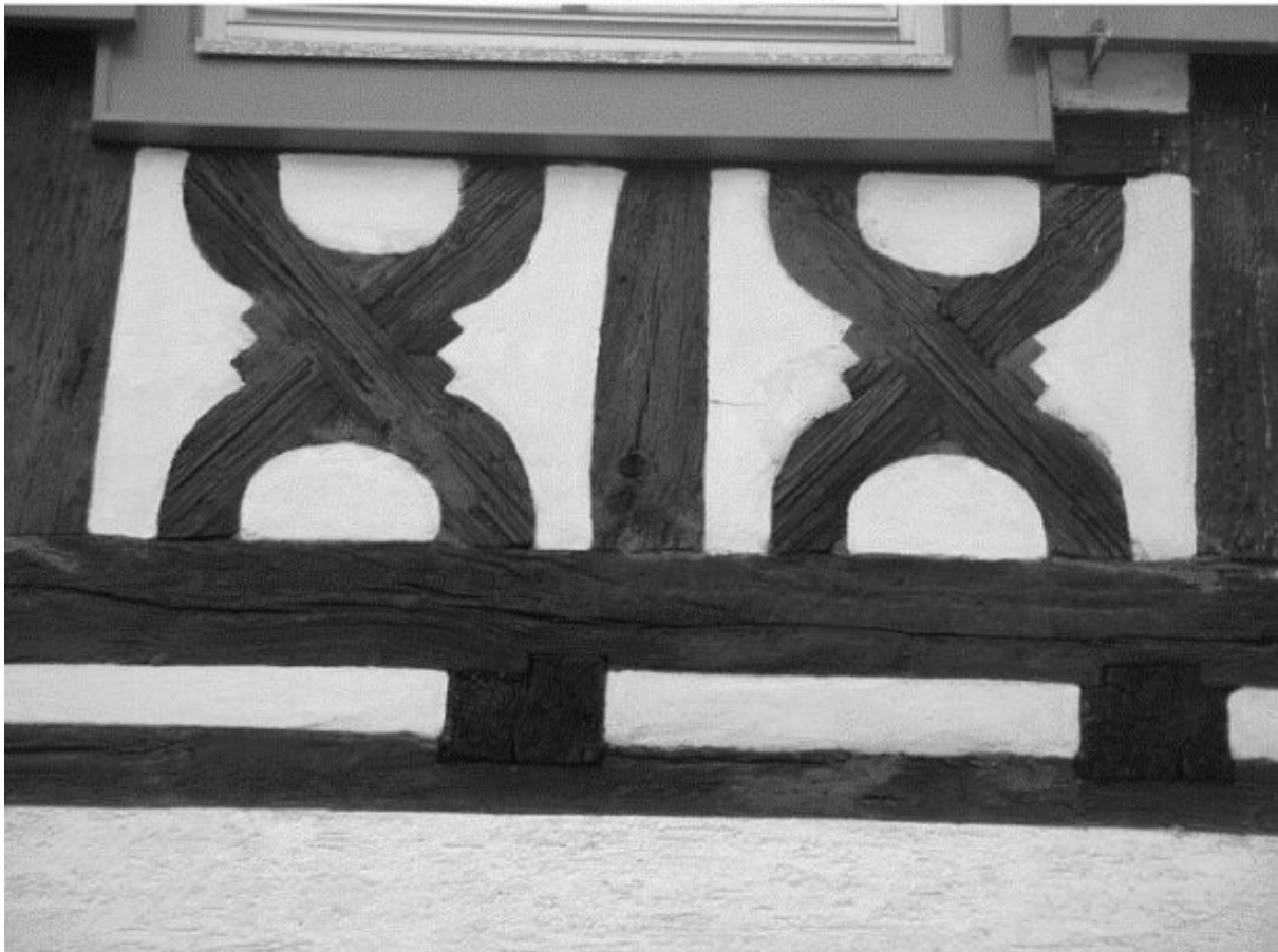
Figure 2-19: Parapet ornaments: top - at a house in Wildungen, built in the middle till end 16 th century. Source: Uhde (1903), Fig. 288 on page 252; bottom - at a house in Durlach. Photo by Michael Kauffmann, 2004.
