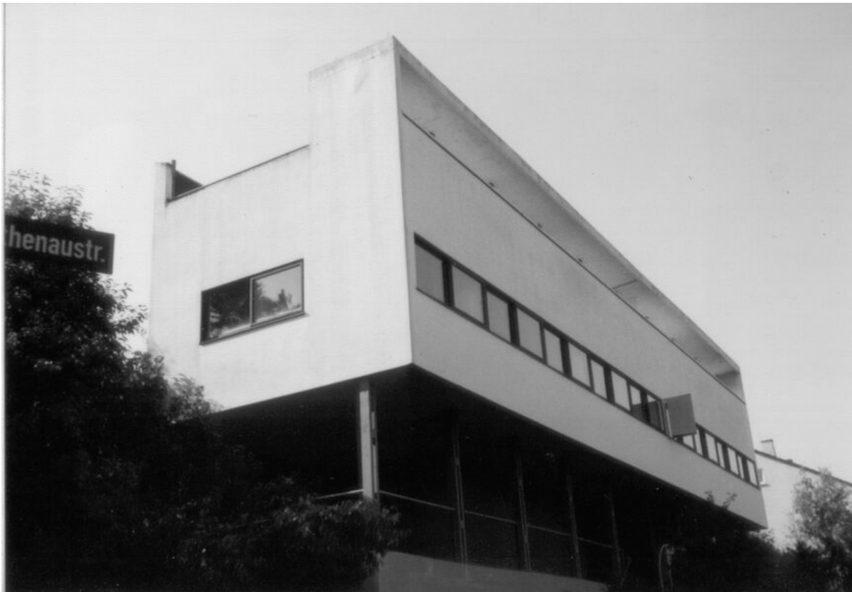
Figure 3-7: A renowned building of this type: Le Corbusier's building in Stuttgart Weissenhof (1927) - a mix of reinforced concrete and metal structure: free standing columns out of metal. Photo: M. Bostenaru, 2002
