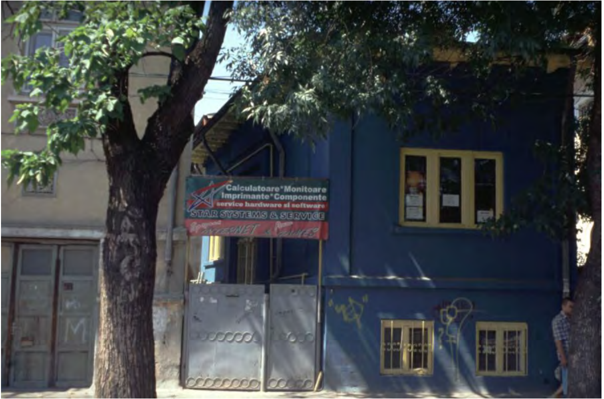
Figure 4-2: Variant of the building with high basement. Photo by Maria Bostenaru, 2002.
