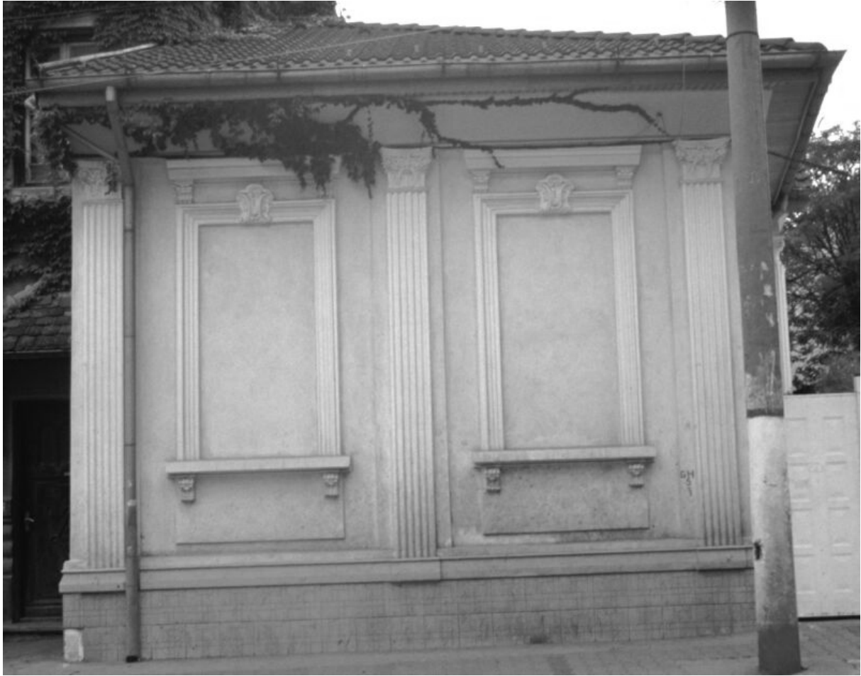
Figure 4-7: Structural modification: Facade with walled-up windows. Photo by Maria Bostenaru, 2002.
