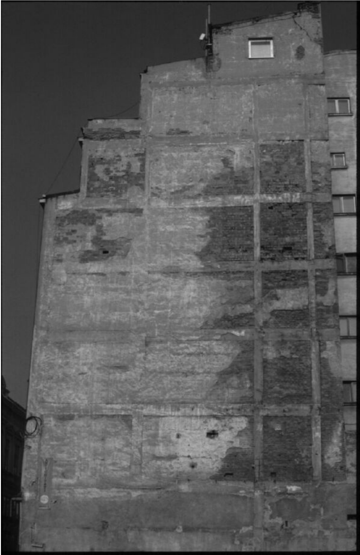
Figure 5-11: Side wall of a typical building (from Bostenaru, 2004)
