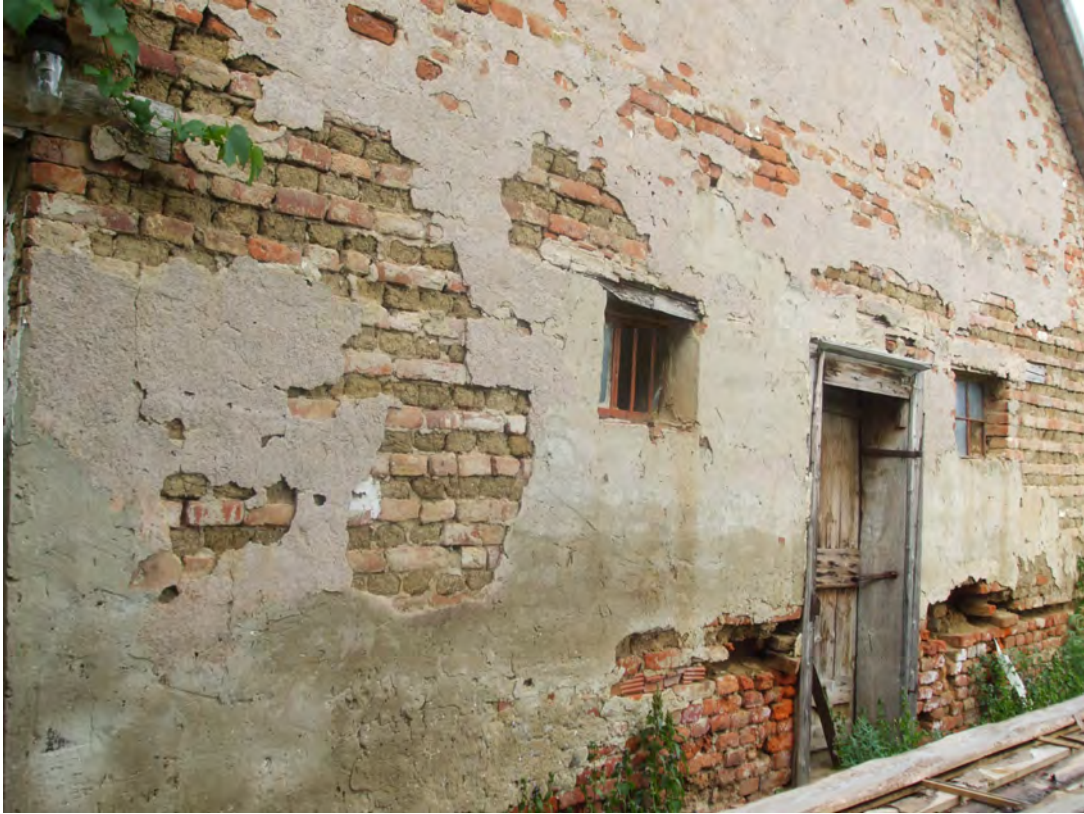
Figure 6-21: Masonry. Photo: Ágota Heinrich, 2009
