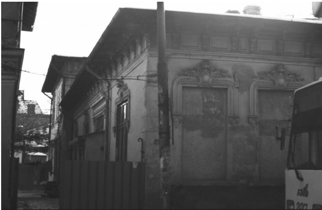
Figure 4-6: Structural modifications: partial upper floor and closed windows to the street. Photo by Maria Bostenaru, 2002.
