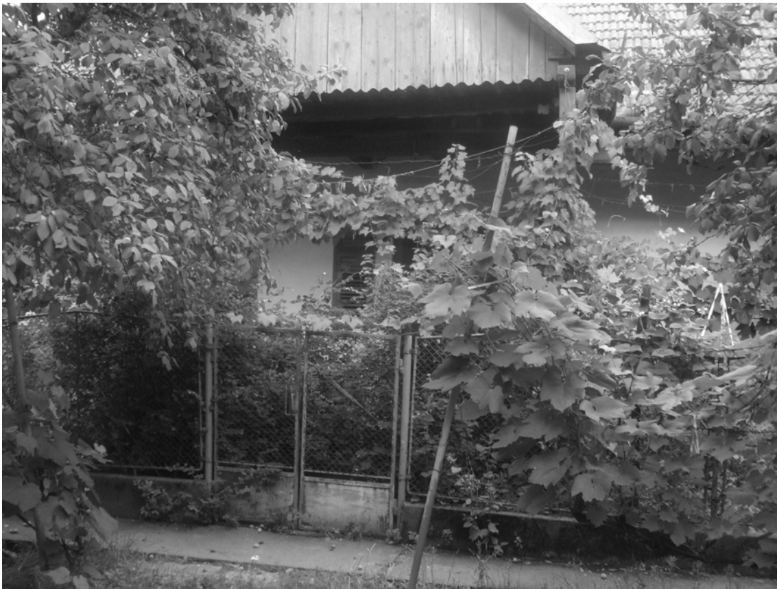
Figure 6-20: End of the roof. Photo by Ágota Heinrich, 2009
