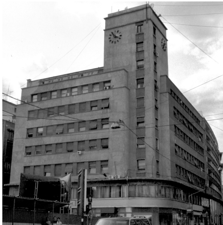
Figure 7-3: Adriatica building, Bucharest (1933). Architect: Rudolf Fränkel. Photo by Maria Bostenaru, 2002.
