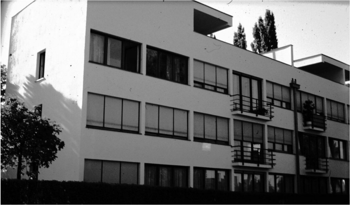
Figure 3-19: Corner detail for a mid-rise building of this type (Stuttgart). Photo by Maria Bostenaru, 2002.
