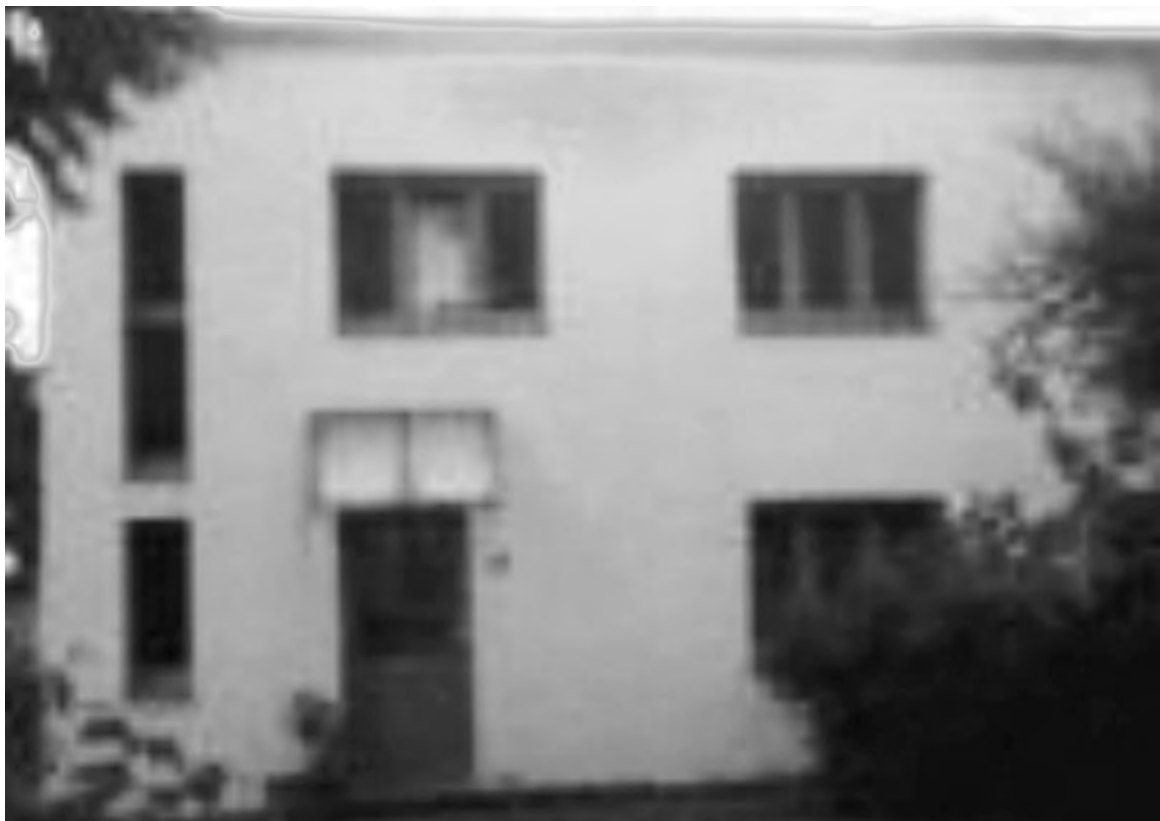
Figure 3-22: Seismic feature (small openings in infill walls): Facade of a low-rise house (Karlsruhe). Photo by Maria Bostenaru, 2004.
