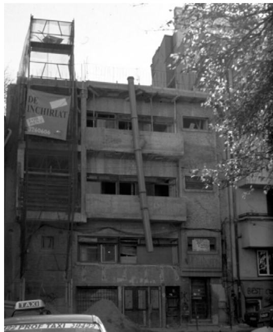
Figure 5-27: Retrofit of such a block of flats. Photo: M. Bostenaru, 2002.
