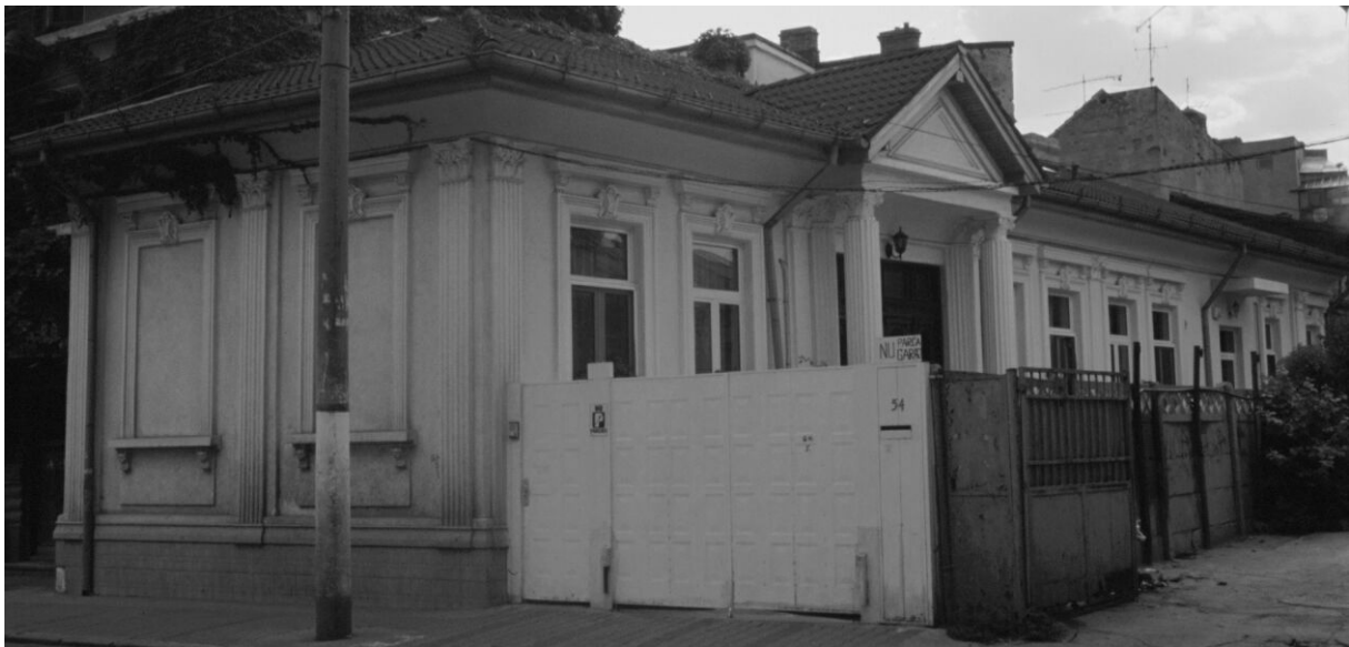
Figure 4-8: Whole view of the building with closed windows to the street (from Bostenaru, 2004, Abb. 2-4 on P. 24)
