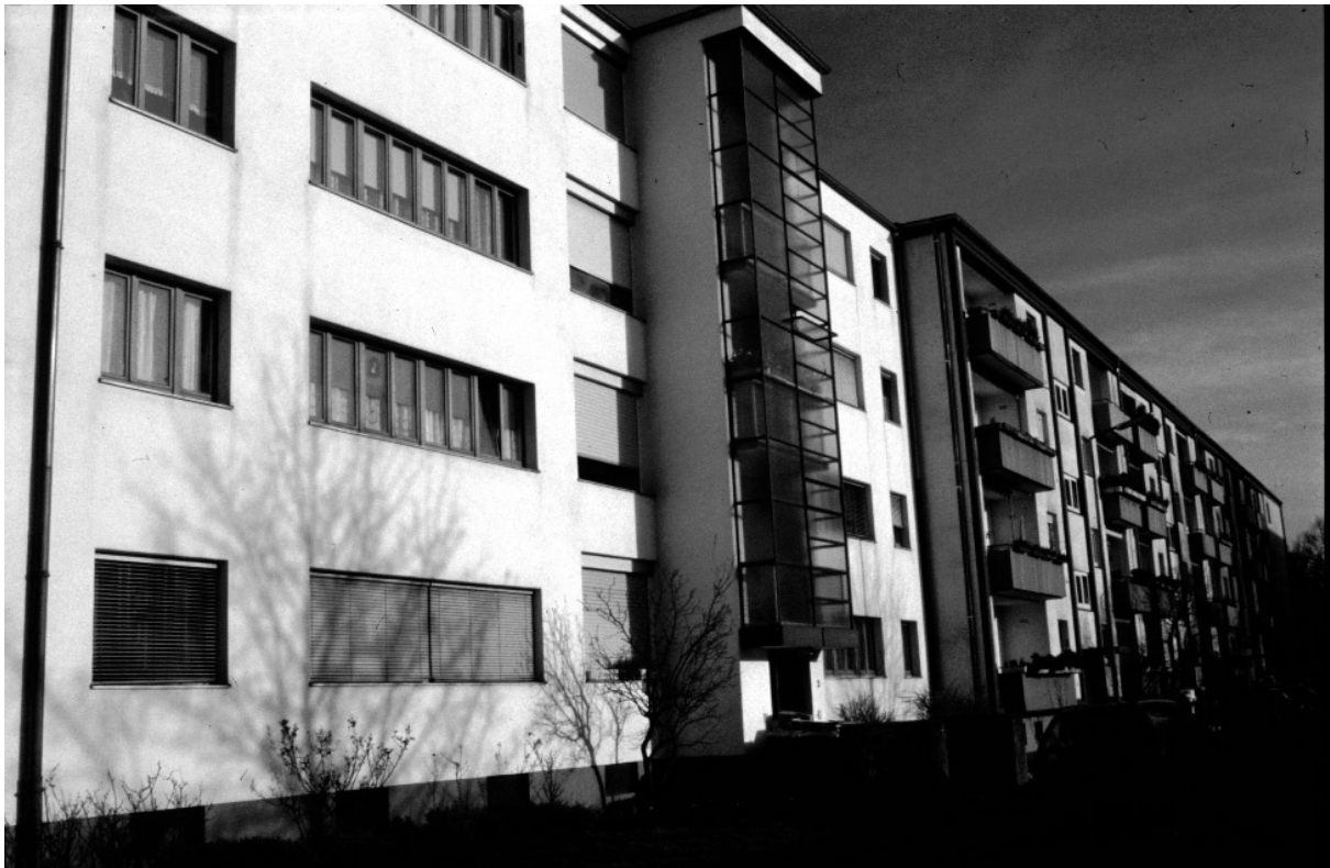
Figure 3-1: Typical photo of a multistorey house of the type (in Karlsruhe; same type to be found in Kassel). Photo: M. Bostenaru, 2004.
