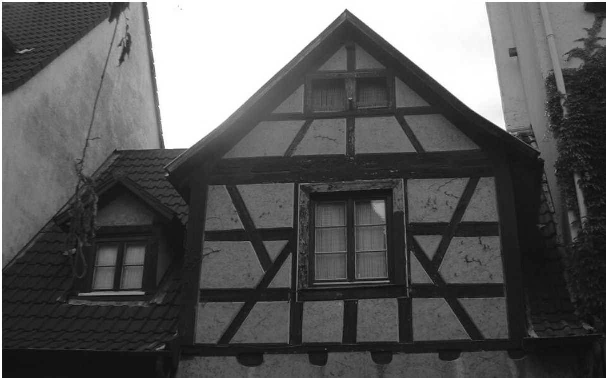
Figure 2-17: Typical window. Photo by Michael Kauffmann, 2004.
