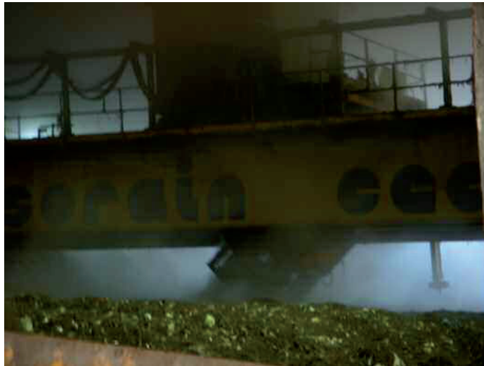
Figure 4 MBT biological ACT section.
