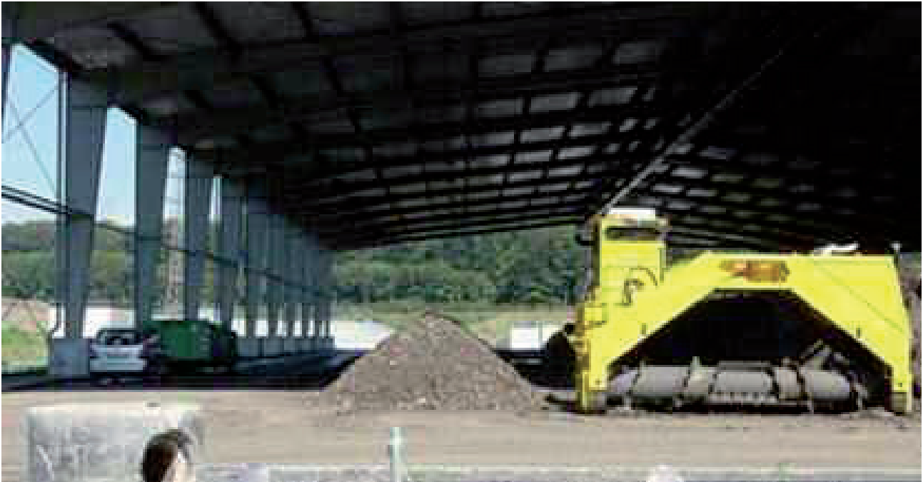
Figure 6: Windrow heap under roof with revolving machine (example)
