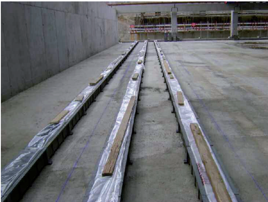
Picture 4: Aeration-floor (under construction)
