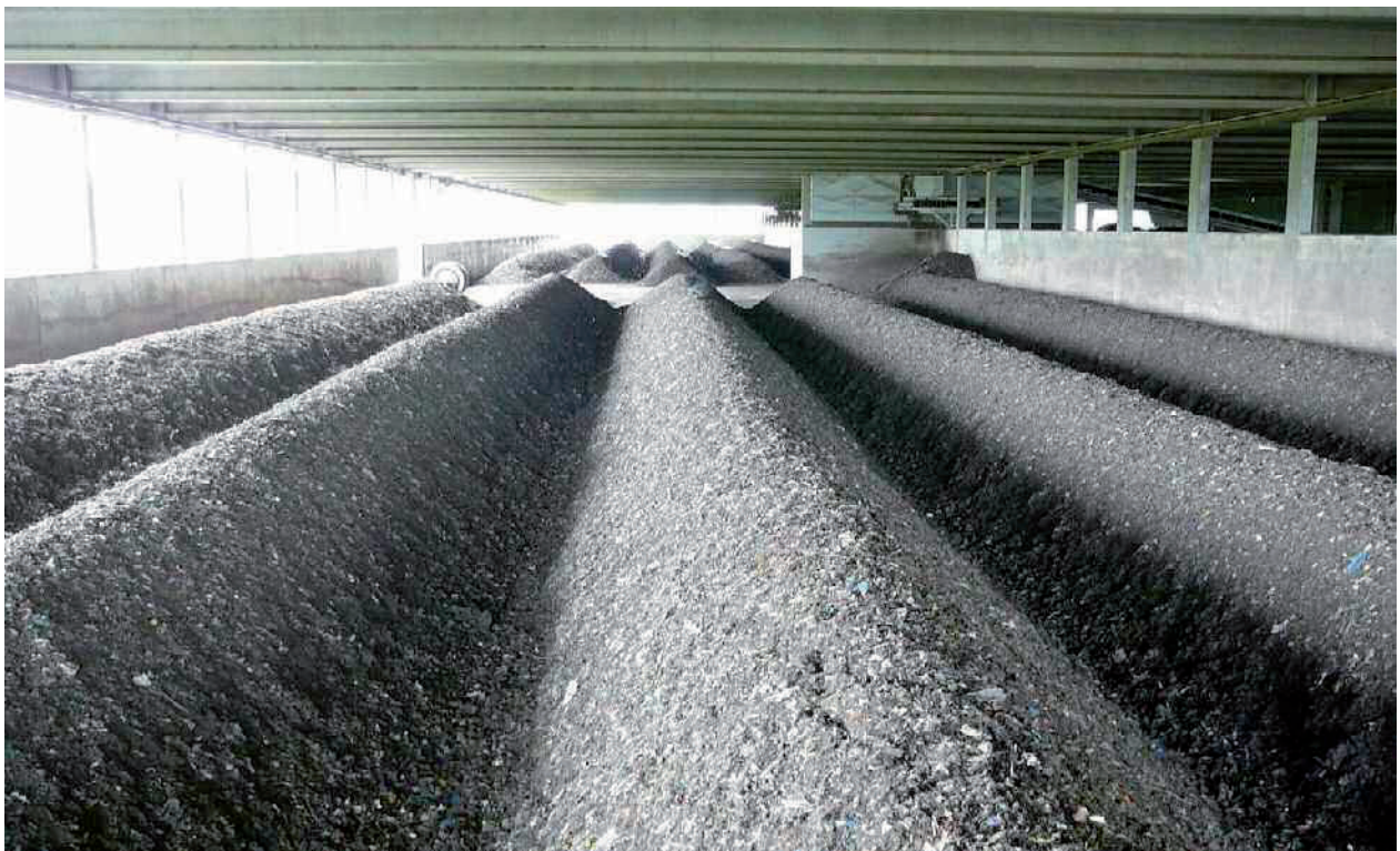
Figure 2 Maturation area of MBT Rosenow
