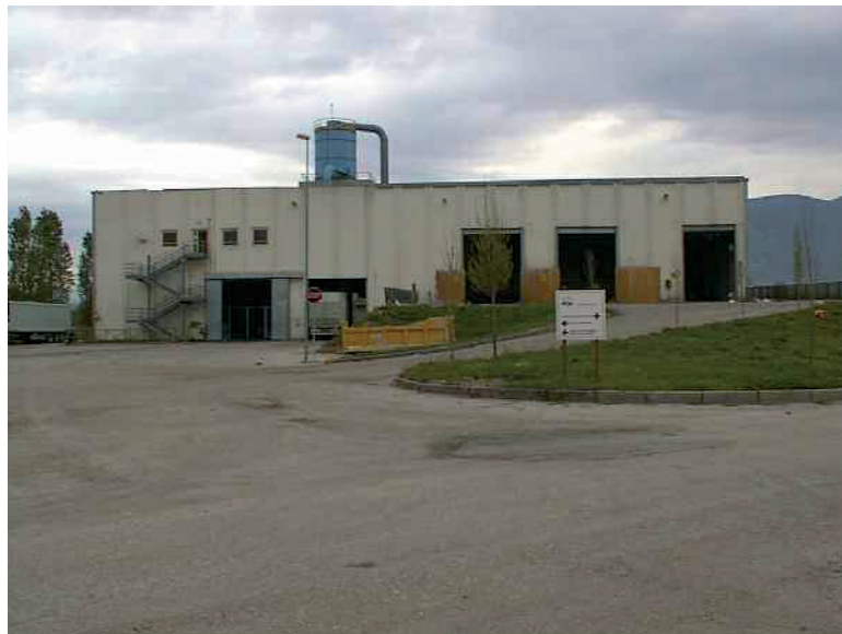
Figure 2 Existing MBT plant.
