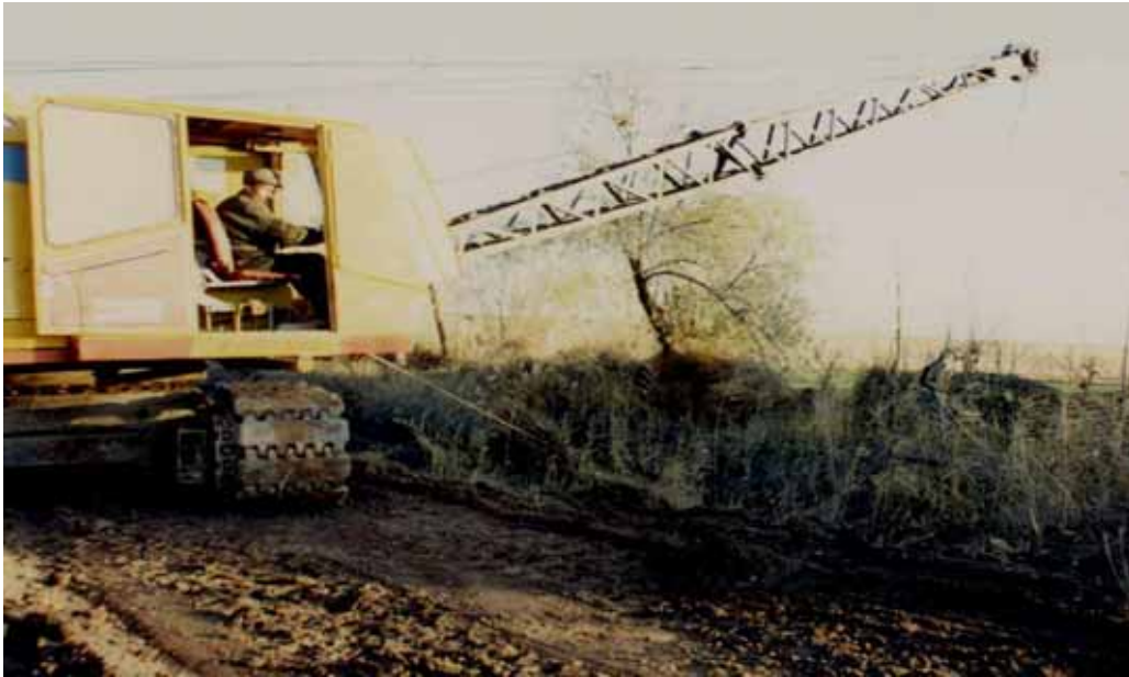
Figure 5.2-3 Cleaning of the canal by excavator (winter, 2002)
