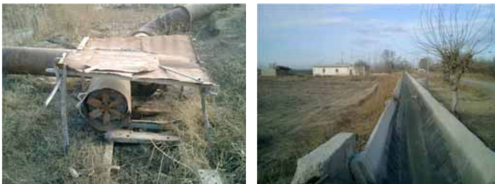
Figure 2.4-3 Condition of irrigation network in Khorezm, 2003 (Own presentation)
