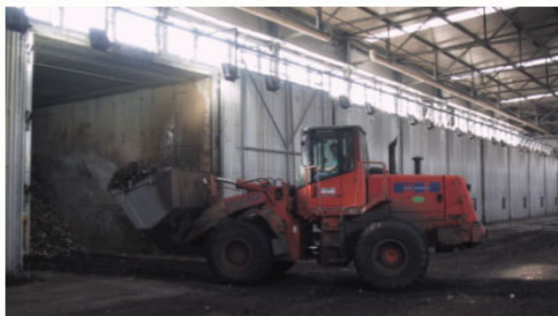
Figure 2: Unloading of a composting tunnel
