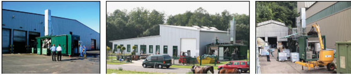
Figure 2: Different locations of the SCHUBIO®-Demonstration Plant
