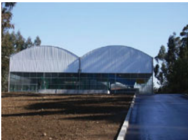
Figure 1 View of the vermicomposting unit
